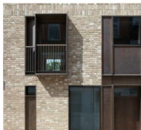
AM3 STEEL BALUSTRADE Flat solid panel vertical steel tube balustrade Colour to match AF2
