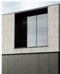
PF7 METAL FINISH TYPE 1 - BLACK Steel metal mounted to large brick openings
