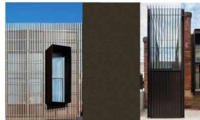
PF17 METAL FINISH TYPE 4 Powder coat finish windows Metal panel cladding Colour powder coat modern/black bronze colour generally
